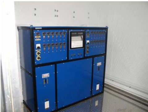
Control Room 24-Way Power Console, washable walls, Diamond Plate Flooring Base Board Heat (optional) Small Desk, A/C unit (optional)
