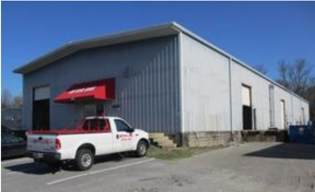
Our Transformer and Welding Machine manufacturing Location (12,000 Sq.ft.) in Chattanooga, TN
